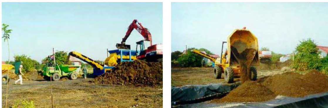
Fig. 1. Soil screening (left) and backfilling in the specially designed cells (right) at the Astra site.
